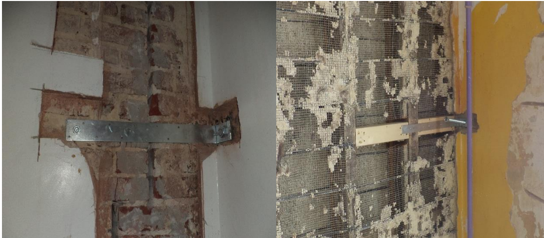
Figure 9. Exterior / Interior Wall Anchorage. (Keast & Hood 2013, with permission from Keast & Hood)
