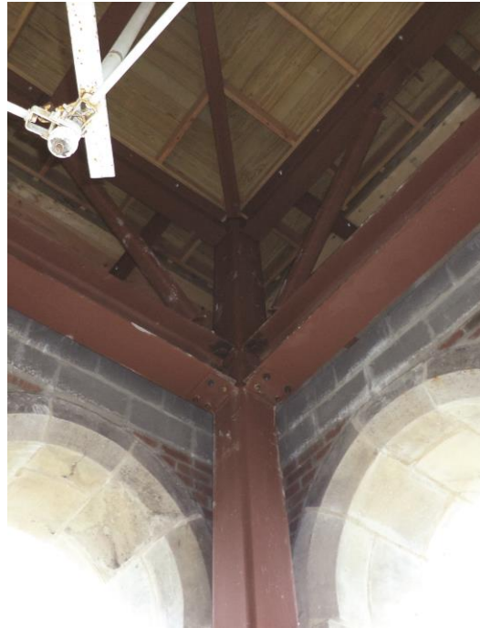
Figure 6. Steel frame from interior.
