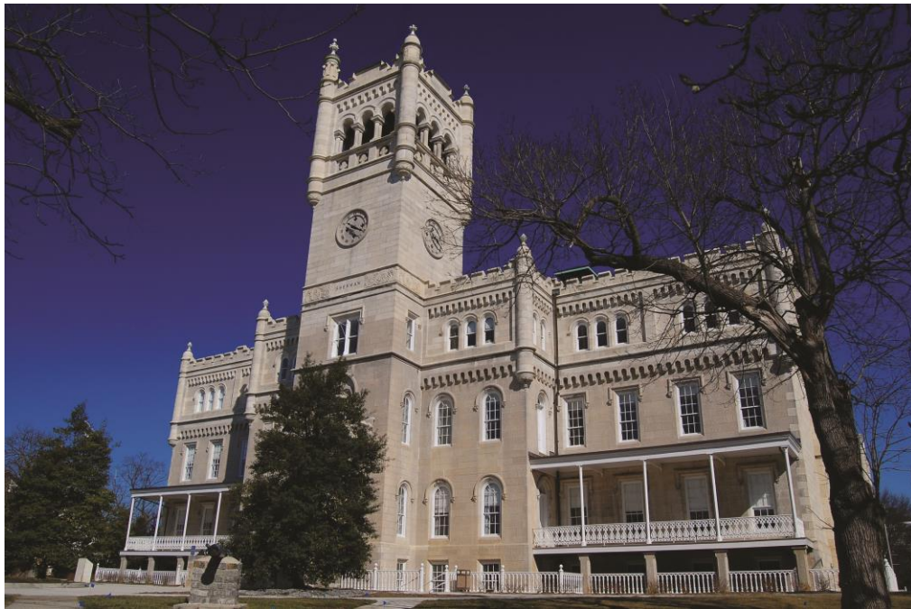
Figure 13. Restored and reinforced Sherman Building. (Keast & Hood 2013, with permission from Keast & Hood)
