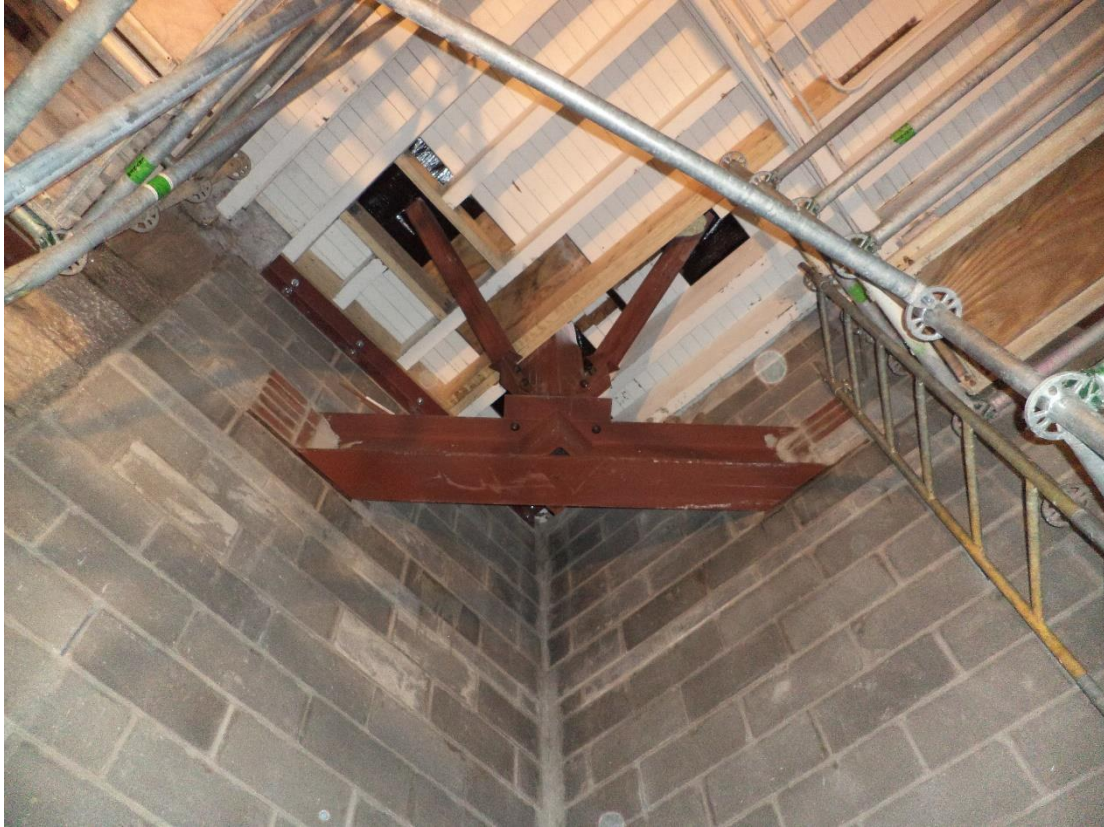
Figure 12. Internal Masonry Shear Wall for Steel Frame. (Keast & Hood 2013, with permission from Keast & Hood)
