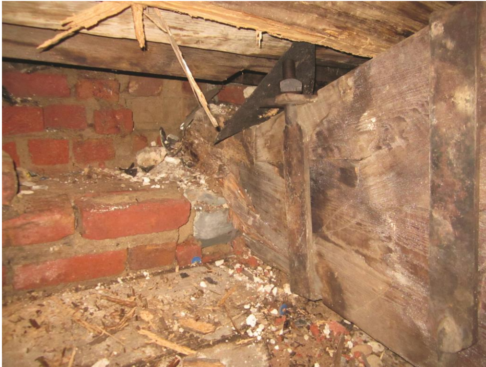
Figure 3. Deterioration in roof truss. (Keast & Hood 2013, with permission from Keast & Hood)
