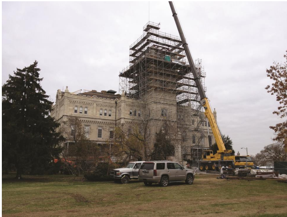
Figure 11. Disassembly of clock tower. (Keast & Hood 2013, with permission from Keast & Hood)
